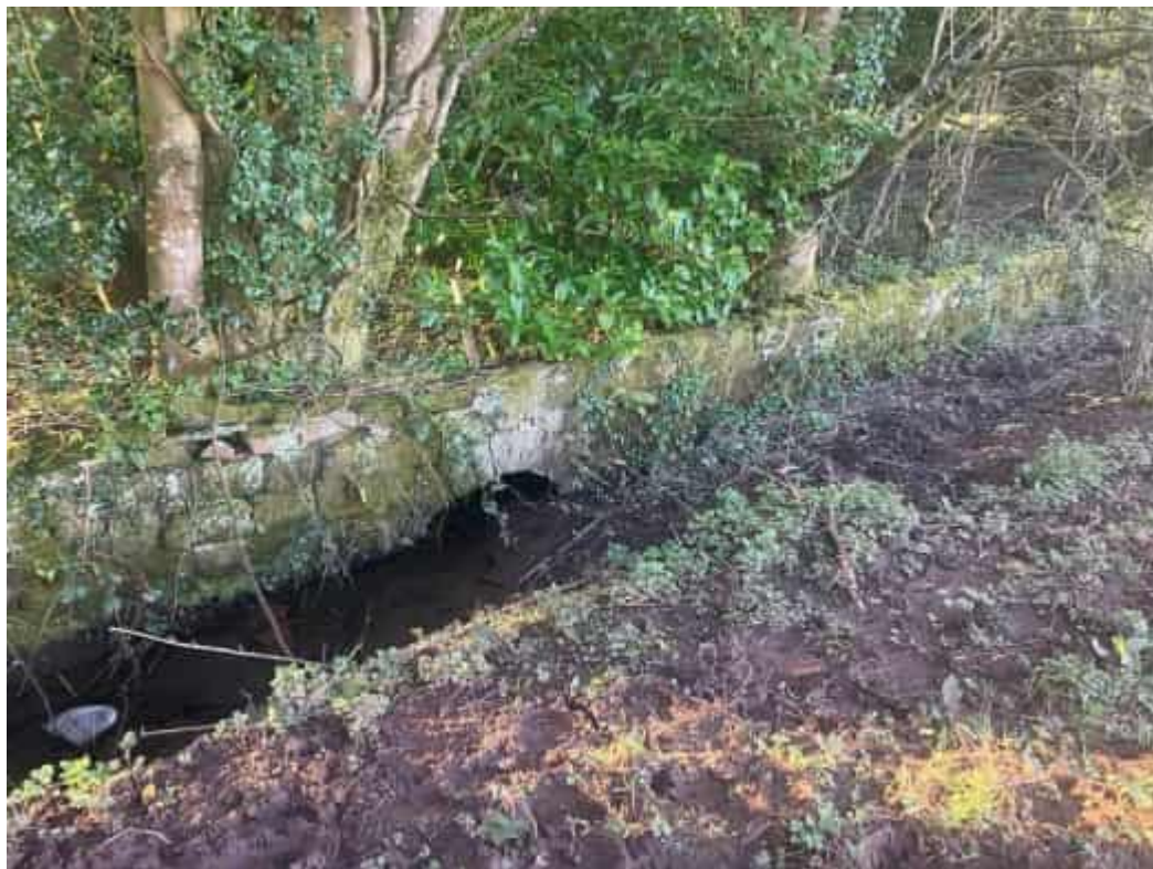
Photo B6 – downstream outfall position of culverted watercourse c. 165m to south-east of site
