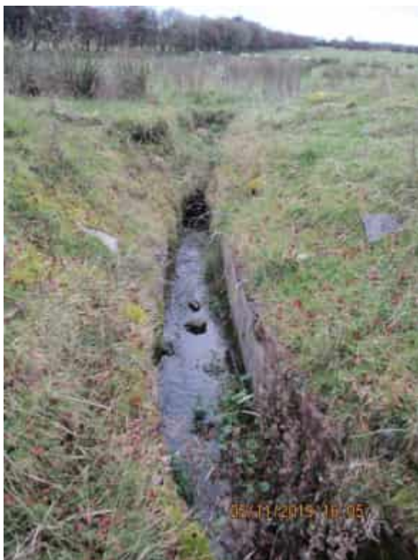
Photo B2 – Section of open watercourse in south-west corner of site looking upstream
