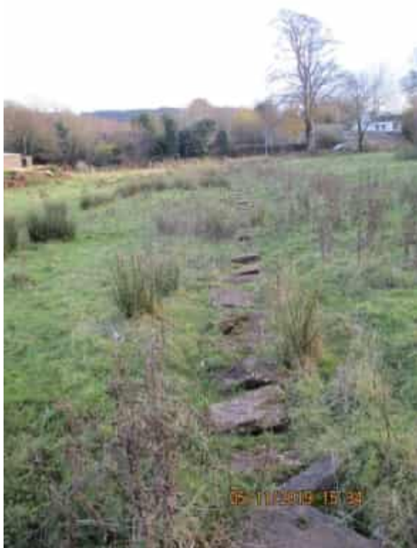
Photo B3 – Section of central culverted watercourse upstream of open section
