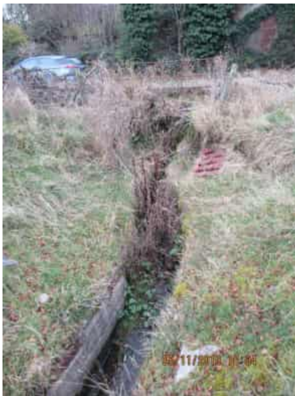
Photo B1 – Section of open watercourse in south-west corner of site looking downstream
