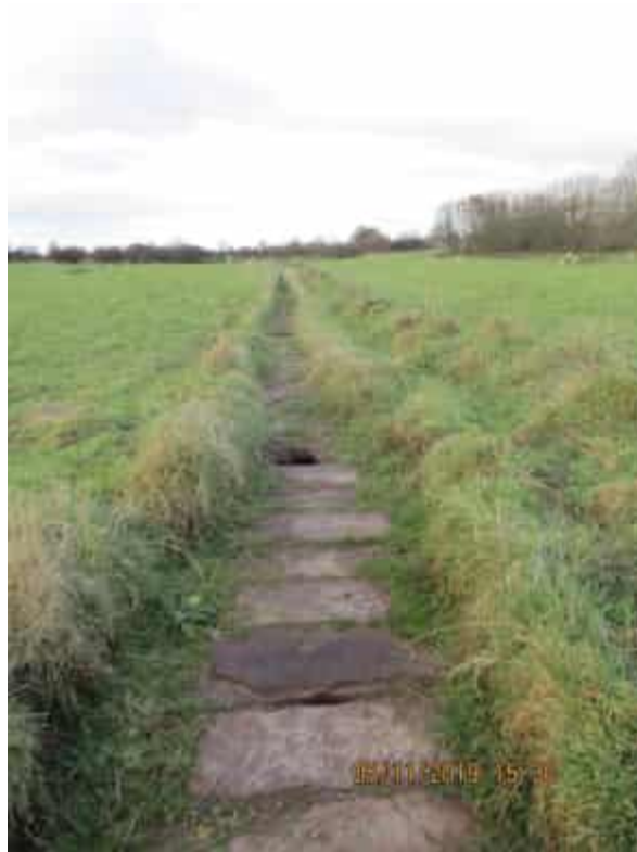
Photo B5 – Western culverted watercourse looking upstream from existing fenceline
